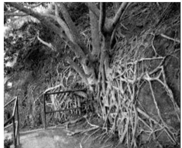
Figure 4E Stabilization of a slope by the root system of a banyan tree, Hawai (source: Google Books Result, http://books.google.com.ng>books )
