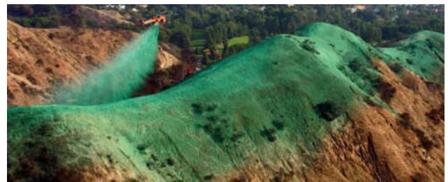
Figure 4C Aerial Hydro-seeding ( http://www.ericksonaircrane.com/hydroseeding.php )
