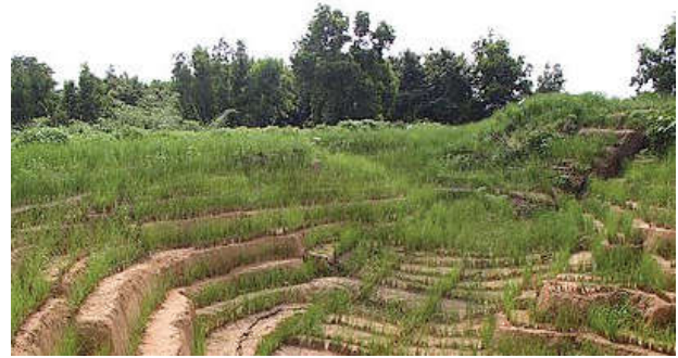
Figure 4D A Vetiver grass system is being used in the Democratic Republic of the Congo for gully control in urban areas and for highway stabilization. These gullies are a major problem in this area and other West African countries ( top ); the same slope now has improved drainage, and the slope has been planted in Vetiver grass ( middle ); this planting of Vetiver grass is about 3 months old.
